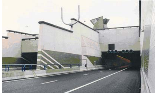
Figure 12.3.2 - Accélérateurs installés aux têtes / Jet fans located in portals
